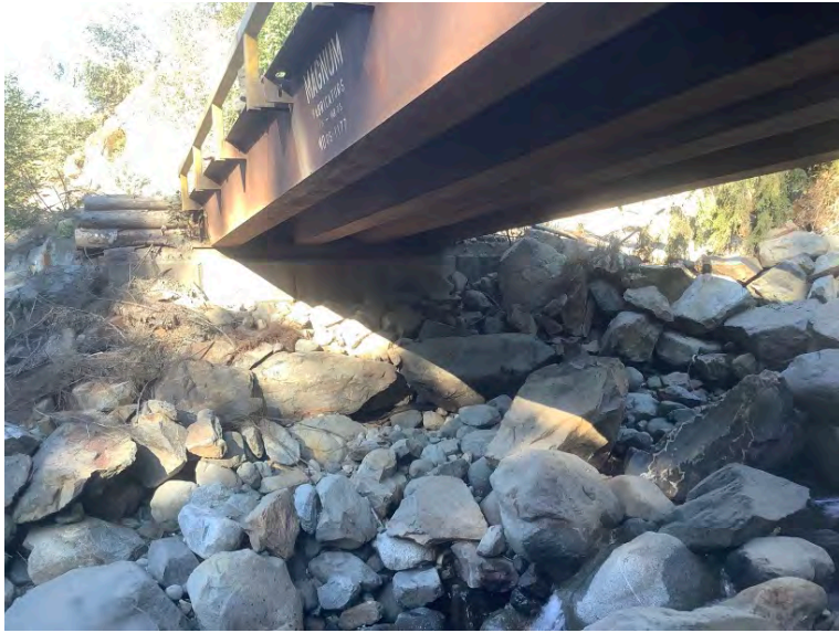
Right Bank Abutment when facing downstream
