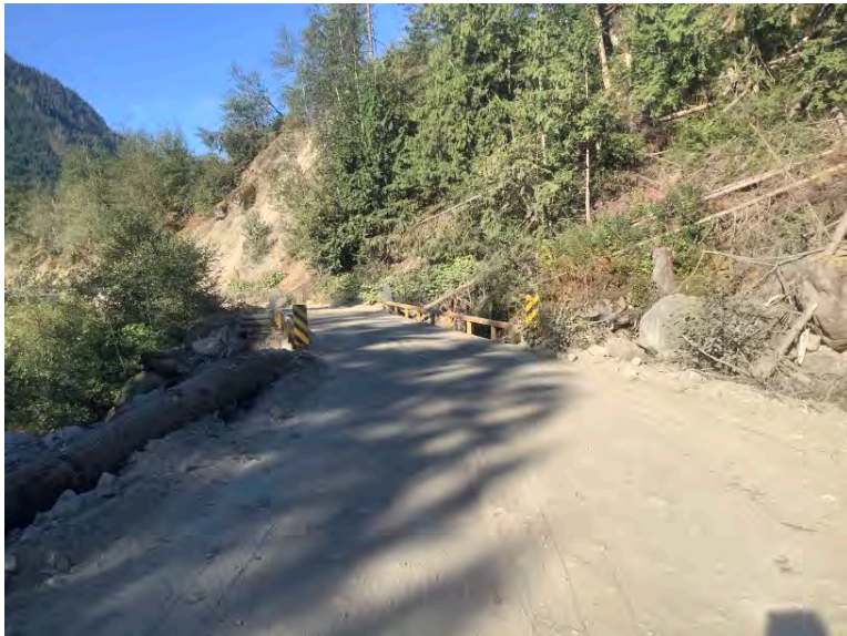
Left Bank Abutment when facing downstream
