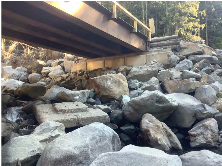
Left Bank Abutment when facing downstream
